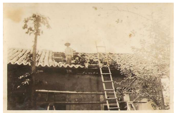
(figure i1.2) - Installing new colonial shingles
